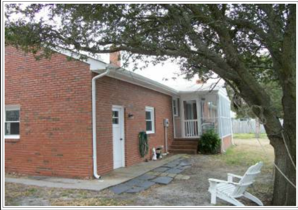
ADDITIONAL REAR VIEW
